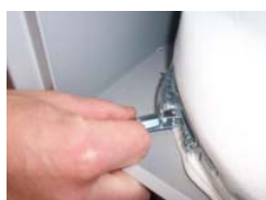
10) Release snap over retaining clip
