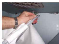
5) Remove rear retaining clip
